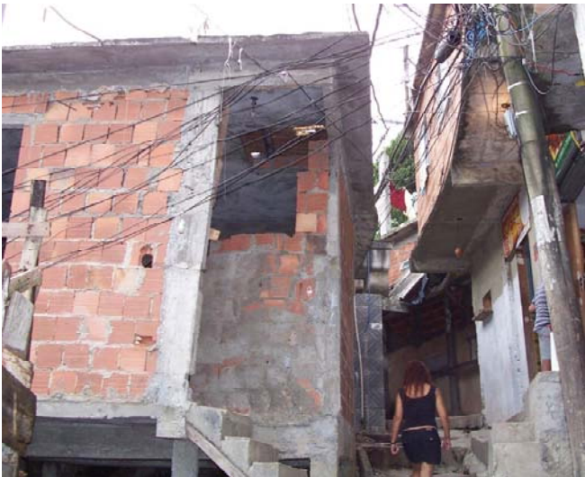
Example of consolidation by upgrading a settlement with more durable materials after property rights have been awarded to the squatter. Fabela Rocinha, Rio de Janeiro, Brazil
